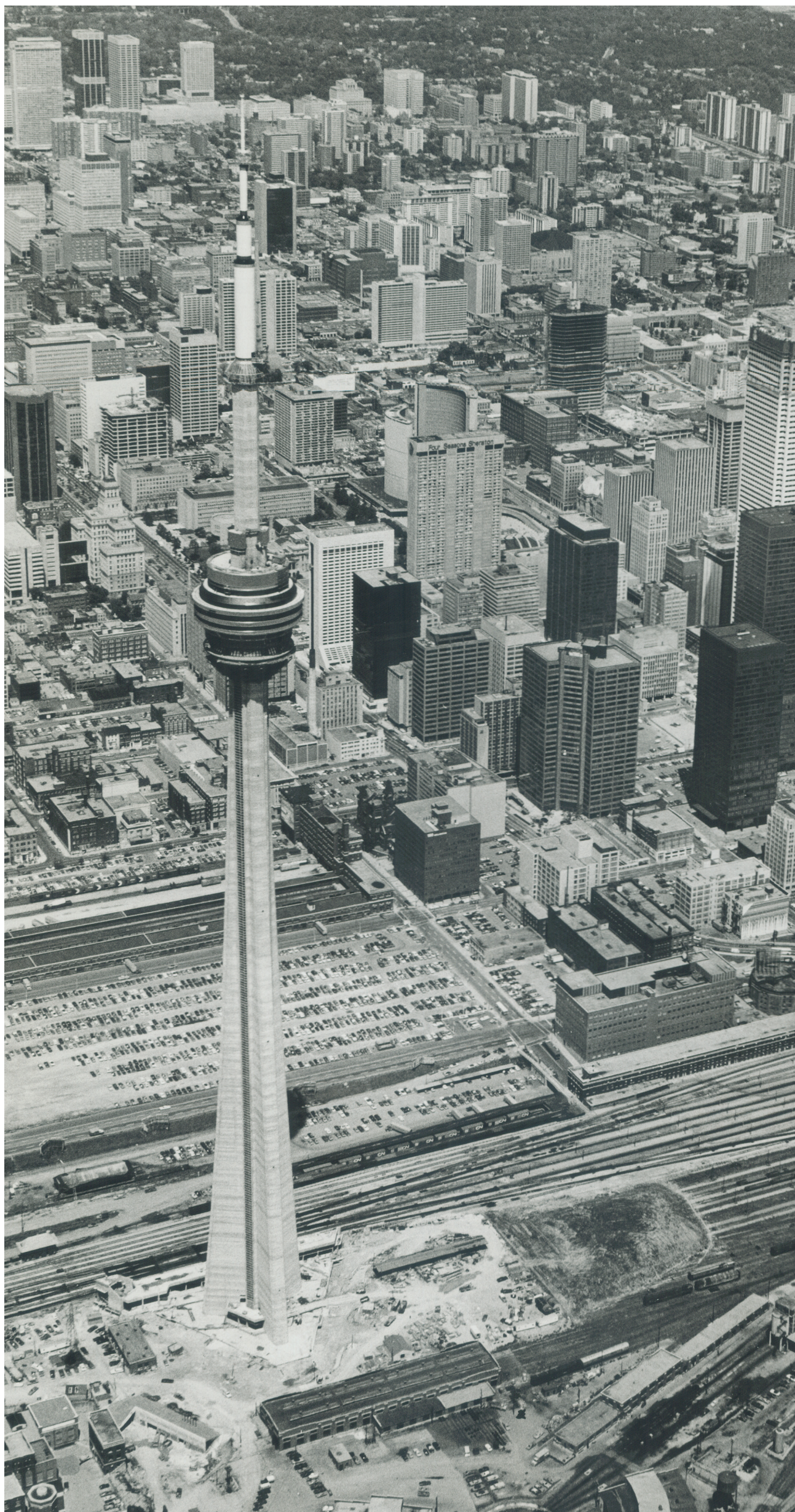
The CN Tower being constructed in downtown Toronto, 1976. Toronto Star, Boris Spremo / Contributor
